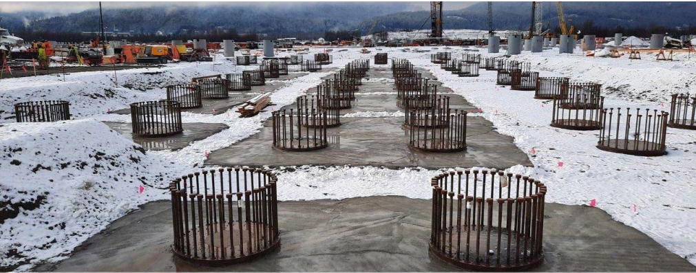
CONCRETE FOUNDATIONS AND PAVING AT LNG FACILITY
