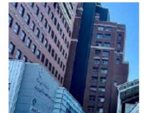
Toronto Western Hospital
