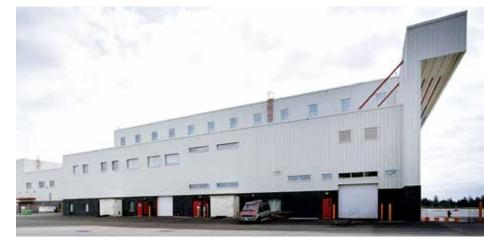
The 8,500-square-metre Fixed Wing Hangar addition was constructed a few years later to accommodate the Buffalo and Hercules aircraft. This was also a steel frame structure with concrete tilt-up panels, and featured specific accommodations for activities related to aircraft operations, barrier-free design, and ammunition security.
