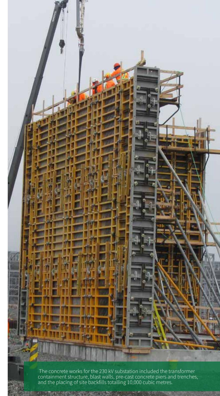
The concrete works for the 230 kV substation included the transformer containment structure, blast walls, pre-cast concrete piers and trenches, and the placing of site backfills totalling 10,000 cubic metres.
