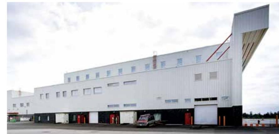
The 8,500-square-metre Fixed Wing Hangar addition was constructed a few years later to accommodate the Buffalo and Hercules aircraft. This was also a steel frame structure with concrete tilt-up panels, and featured specific accommodations for activities related to aircraft operations, barrier-free design, and ammunition security.
