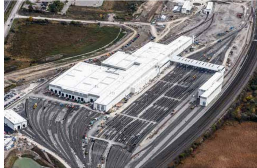
The facility achieved LEED® Gold certification through measures such as the installation of reflective roof materials to limit solar radiation, maximization of natural light within the main building, diversion and storage of rainwater to lower the impact on municipal infrastructure and for use in the wash stations and washrooms, the creation of dedicated car pool parking locations, and the provision of electric car charging stations.
