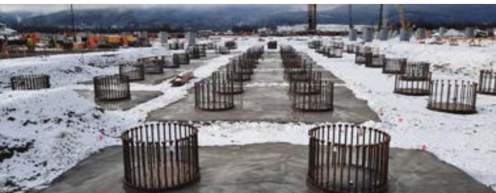
CONCRETE FOUNDATIONS AND PAVING AT LNG FACILITY
