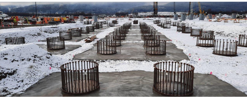
CONCRETE FOUNDATIONS AND PAVING AT LNG FACILITY
