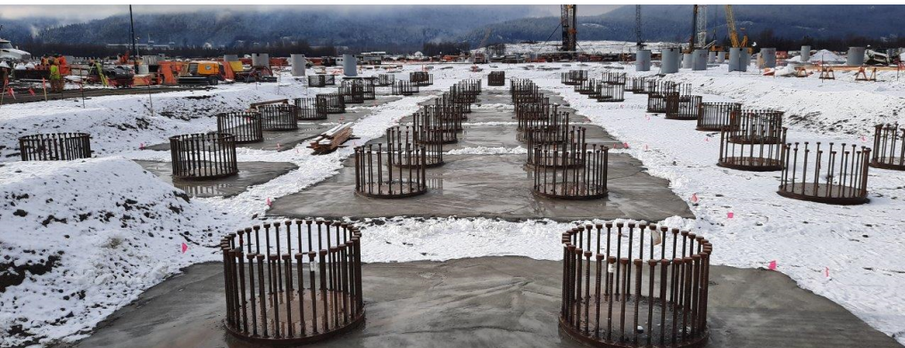
CONCRETE FOUNDATIONS AND PAVING AT LNG FACILITY
