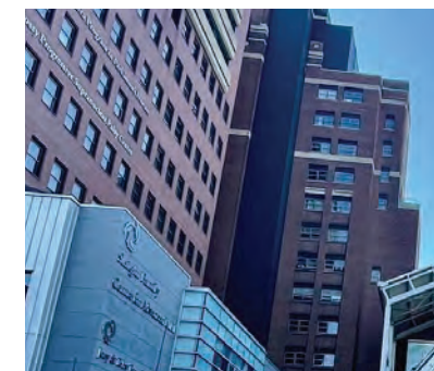
Toronto Western Hospital
