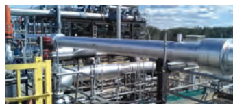
Insulation and Cladding
