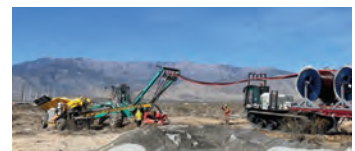
One Pass Trenching / Utilities Installations
