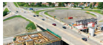
Horizontal Civil Works
